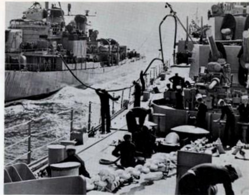
"That's well"--the signal that fueling hose is properly aligned
